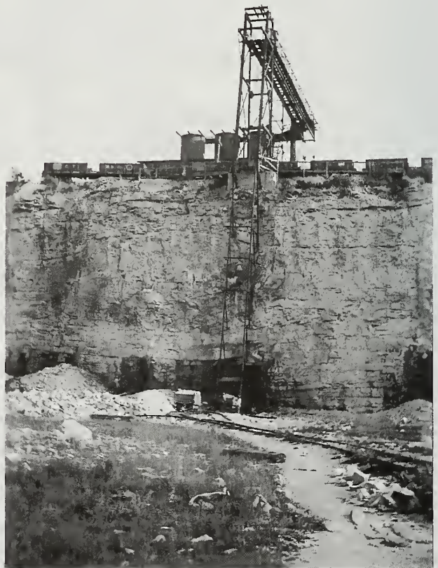
Figure 11 South wall of Brownell Improvement Company quarry (near center of present South Pit and since removed) showing hoist to steel lime kilns in 1907. About 80 feet (25 m) of interreef strata are visible. Irregular bedding near center of wall may be a megaclast or fore-reef that was located about the same distance from the main reef as features in west wall of present South Pit. (Photo by E. F. Burchard, No. 432, U. S. Geological Survey Library)
